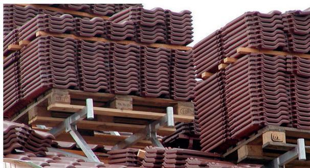
Maximale Last 5 kN (500 kg) pro Plattform = 10 kN pro Paar.
